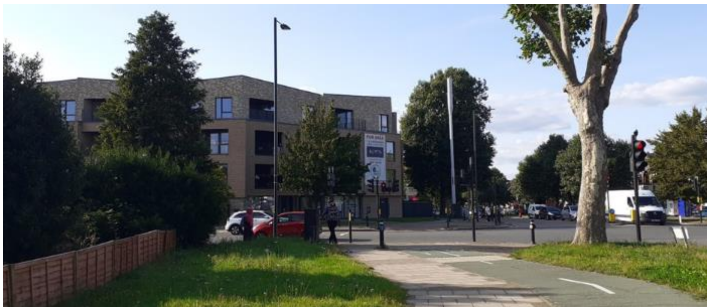
Recent photos of the Matrix development, opposite application site
